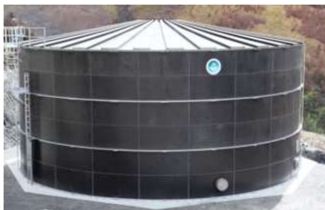
Figure 5: Example of the overall shape of the reservoir tanks
