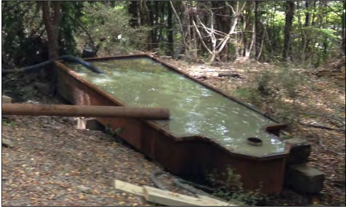
Figure 5: Water sump used for recycling and sediment collection
