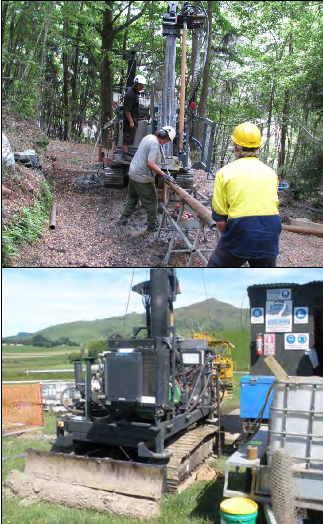
Figure 4: Drill Rig, which will be located on wooden platform (except within Judah Mine area), along with core and water and fuel containers.
