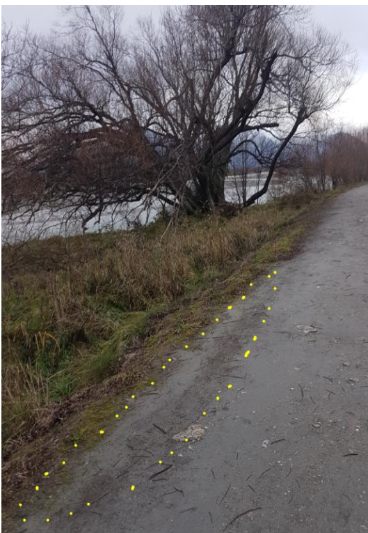
Figure 7 - Indicative surface slumping of the embankment crest
